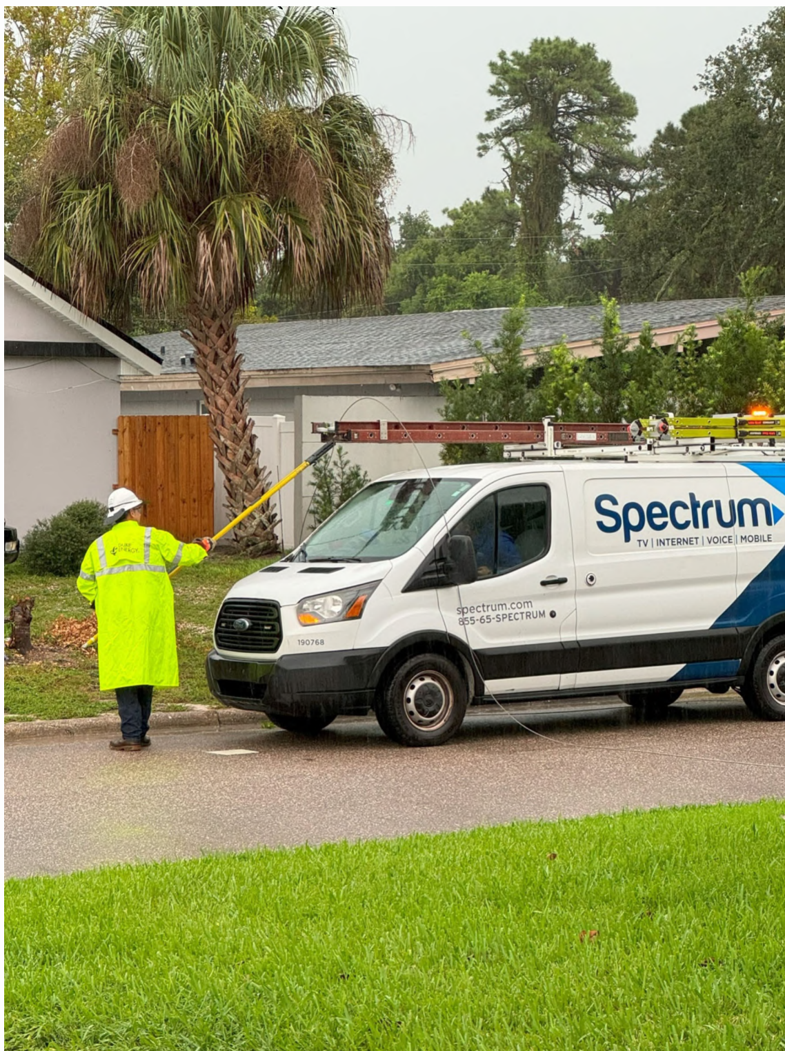
Duke Energy Worker Removing Neutral Wire from Spectrum Vehicle
