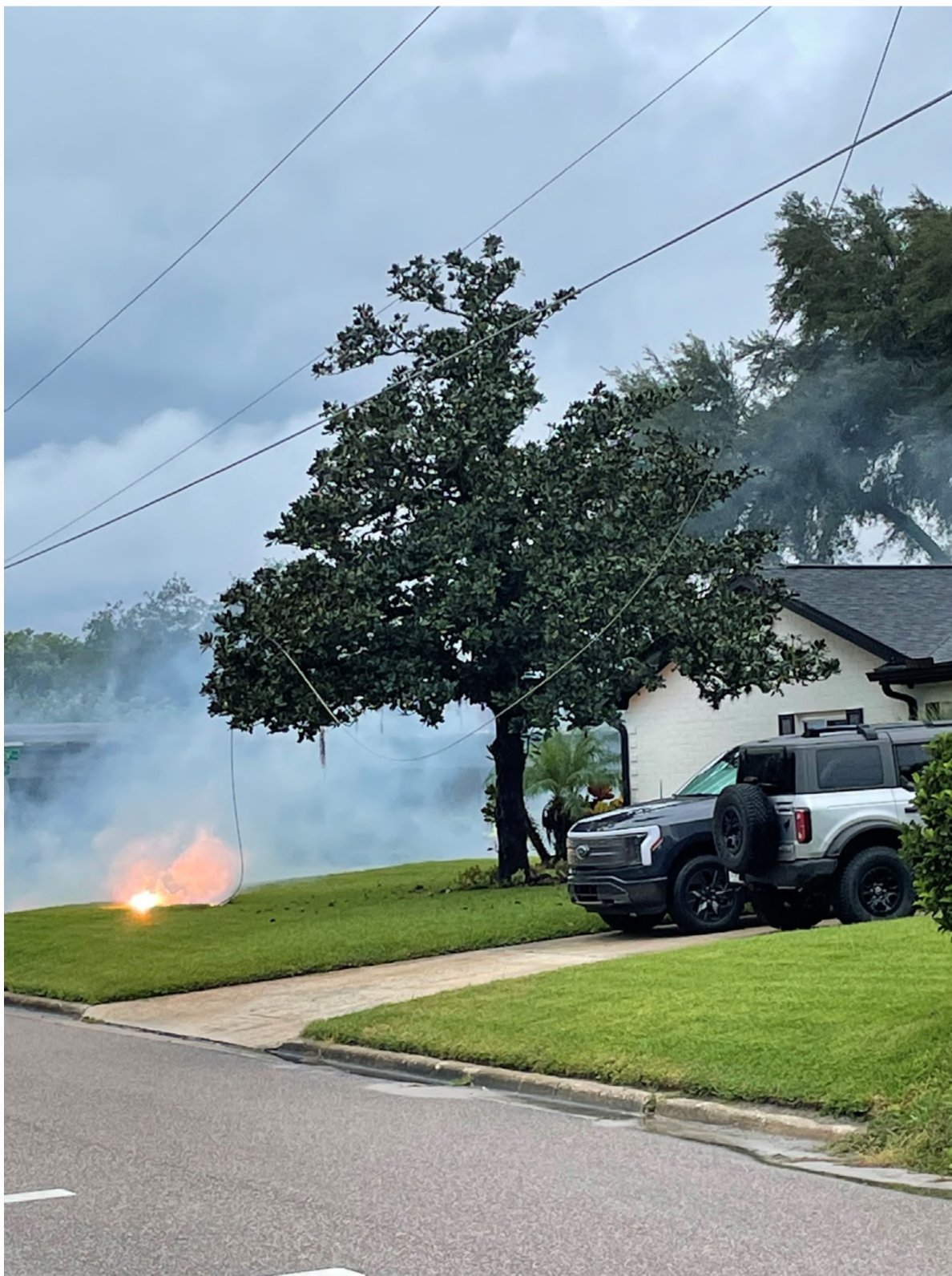
Power Line Burning Trench in Yard and in Contact With Magnolia Tree
