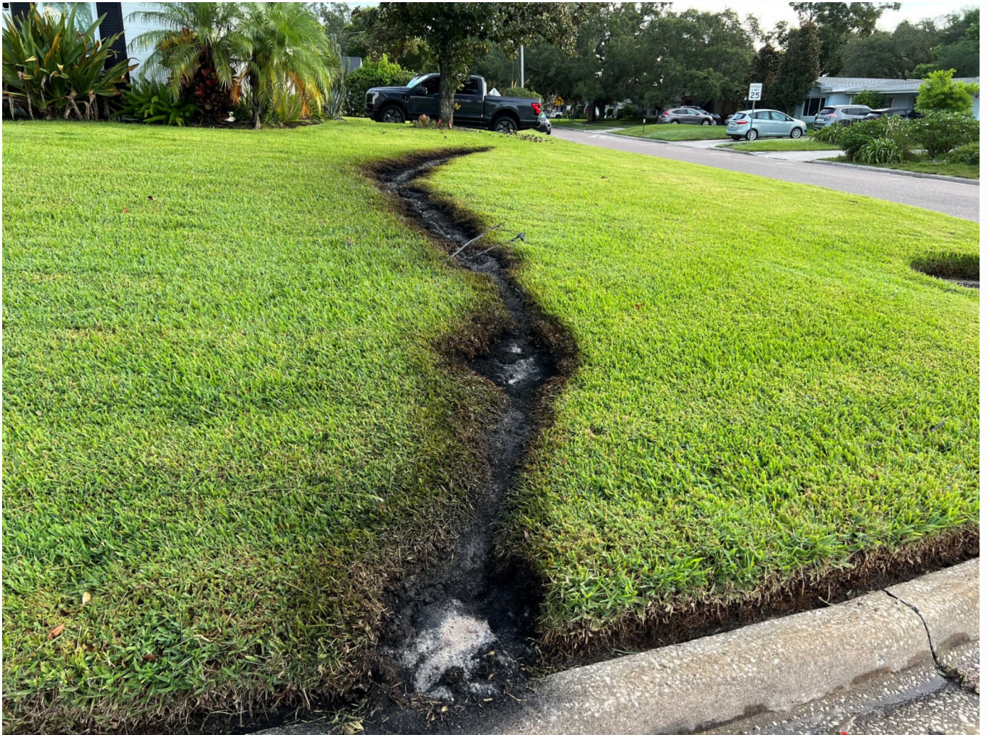
Trench Burned by Power Line
