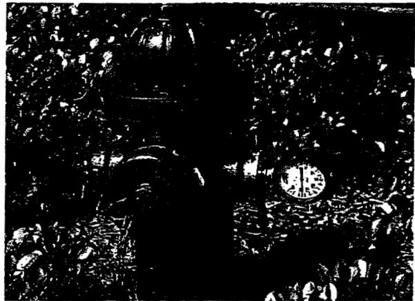
On-site Fire System Pressure Reading 135 PSI
