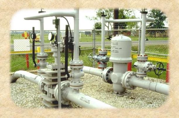
Each valve that might be required during an emergency must be inspected and partially operated at least once each calendar year not to exceed 15 months.
