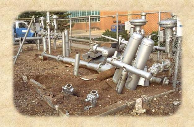
\* Each valve, necessary for safe operation of a distribution system, must be checked and serviced once each calendar year, not to exceed 15 months.
