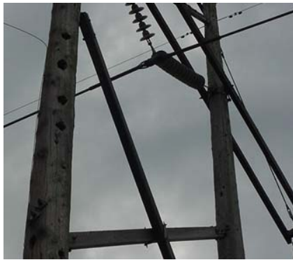
State 5 WoodPecker Holes (with large internal cavity)
