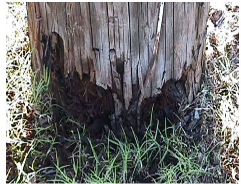
State 5 Groundline Pole Decay
