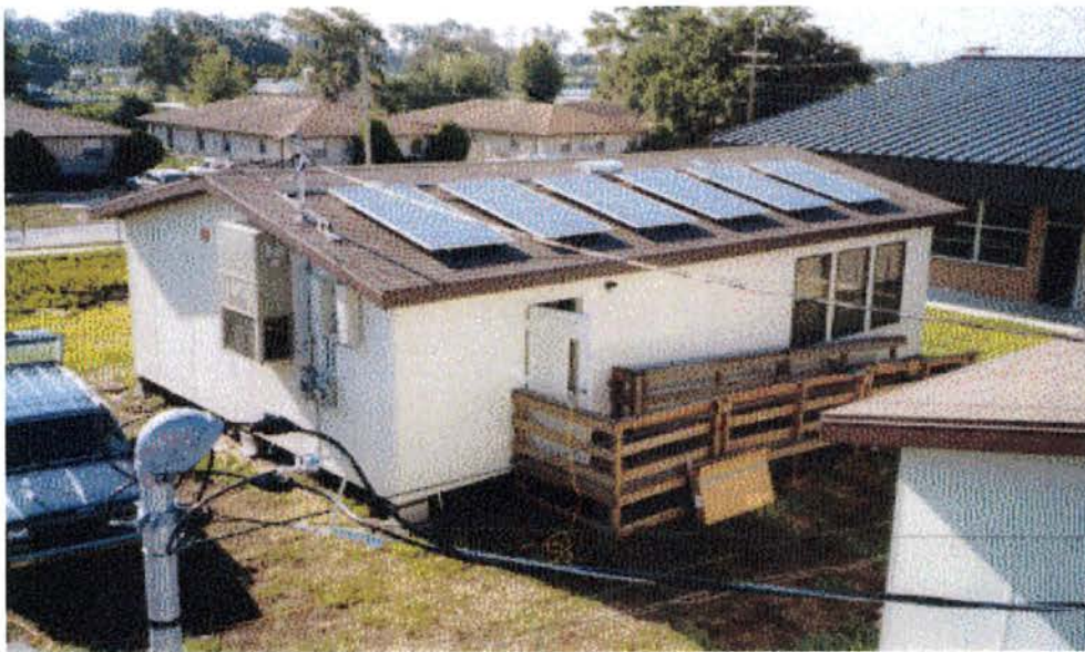
Figure 4-2 Portable Classroom Topped by PV Panels
