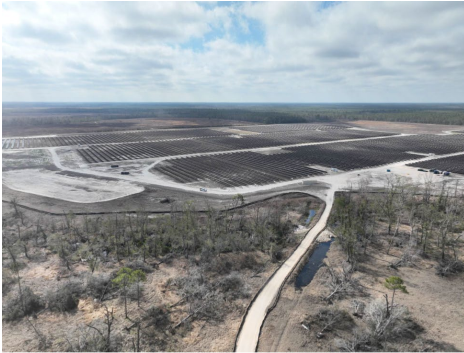
FIGURE 3.2 Sundance Solar Power Plant
