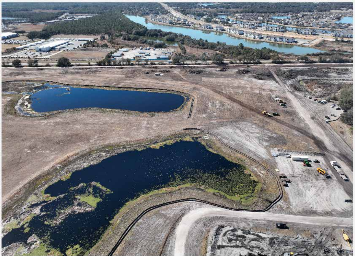
Figure 7-6: Edge Solar - Project Site under construction
